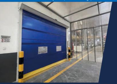
The maximum service life of conventional parts of this product is 500,000 times, with the functions of dividing plant area, noise reduction and dust prevention, wind resistance and insect prevention. Suitable for pharmaceutical and food factory entrances and cold storage area and other building areas. By preventing external factors from disturbing the working environment and improving the working environment, the purpose of reducing energy consumption and improving product quality.
